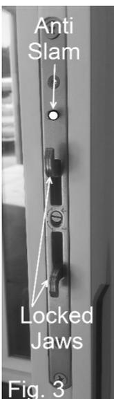
While pressing the anti-slam button on the lock, put the lock in the locked position. (Fig. 3) Using a pencil, mark the height location of the locked jaws. While centering in the pocket, secure the keeper. Having solid shims behind the keeper is critical for years of service free operation. Don't forget to unlock the lock. Test the operation of the lock. Remember that the end users experience with the door will come from the ease of locking & unlocking, as well as the sliding of the door.
